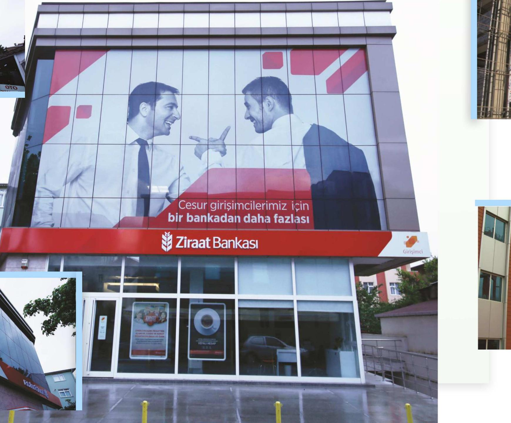
E N | Aluminium structural silicone facade system, aluminium, thermique insulation and joinery, wall covered by composit panels in aluminium.
