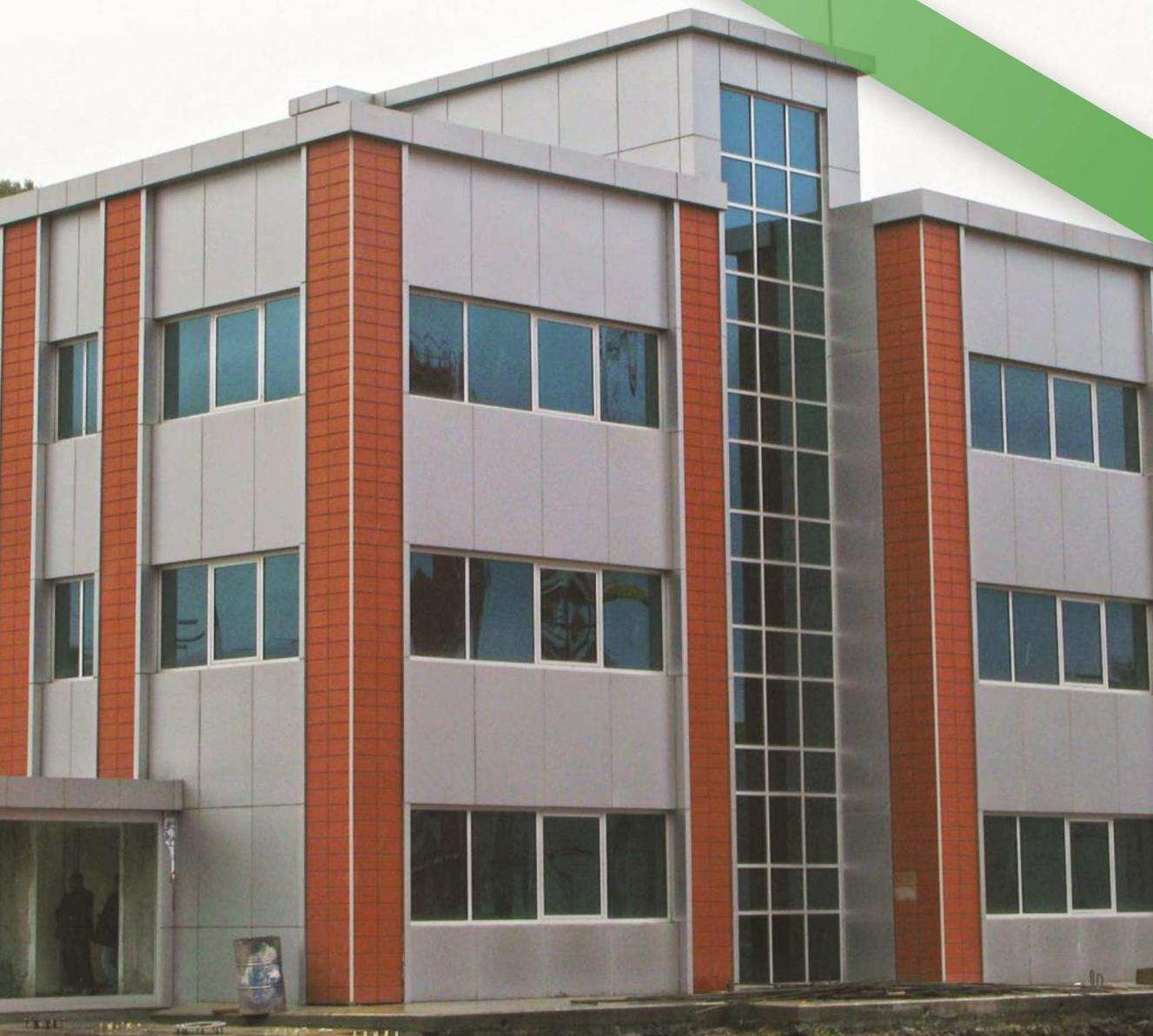
E N | aluminium thermique insulation and joinery, wall covered by composit panels in aluminium and stone, otomatic door system, curtain wall transoms and mullion
